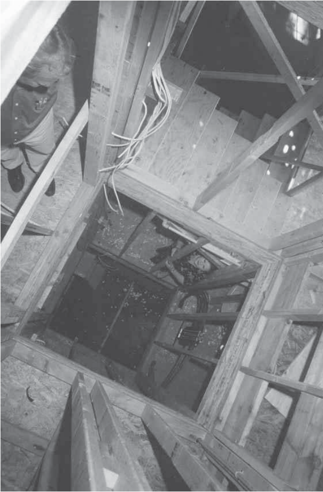
Figure 3. Two floors of stacked closets framed for future elevator shaft.
